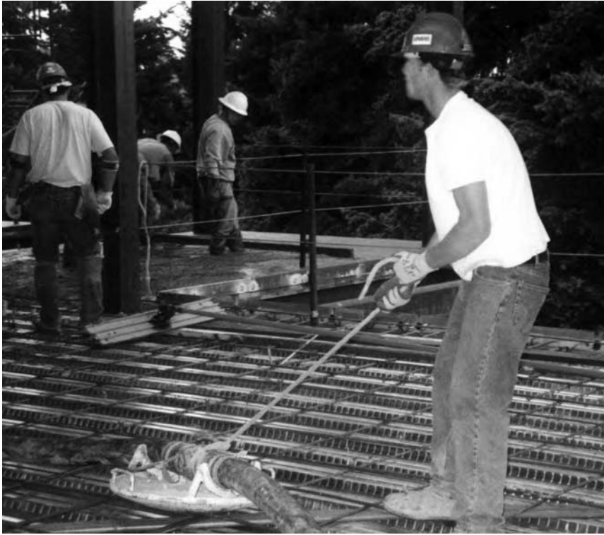
FIGURE 50.3 Steel skid plates under a concrete hose junction. (From Hess et al. Elsevier, 2003, With permission.)
