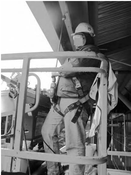
FIGURE 50.7 Drill extension to modify posture.
