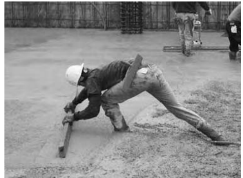
FIGURE 50.4 Leveling concrete manual screeding.
