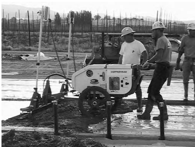
FIGURE 50.5 Leveling concrete by laser screeding.
