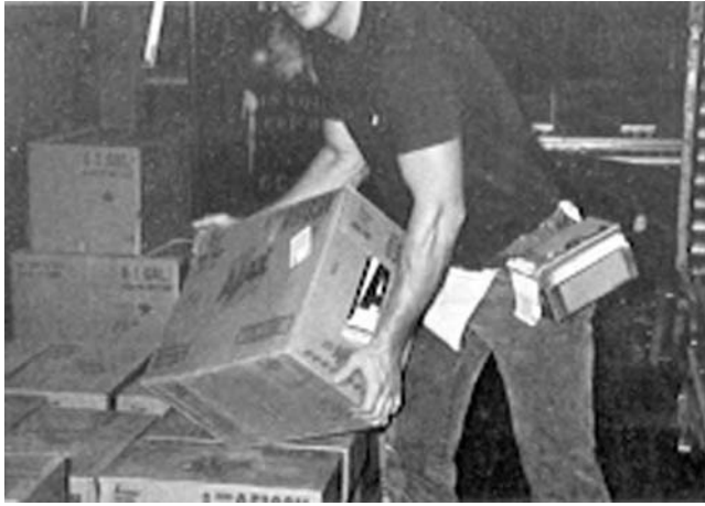
FIGURE 45.24 A waist-held sticker dispenser, used to free up both hands for order selecting.
